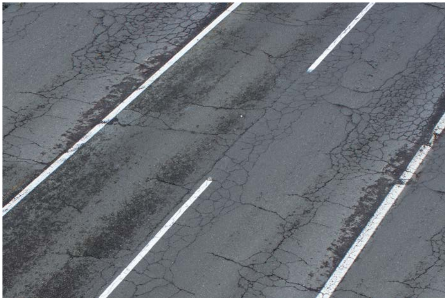
Figure 60. A cracked road surface due to too hard an asphalt binder being used. Another common problem (not shown here) is the rutting seen when too soft a binder is used.
